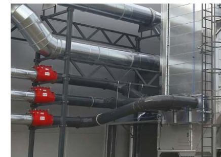
The installation of B-FLAP I on the exhaust duct
