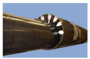
Fix plastic holders with clip on the inner wall of the casing pipe. Cut to suitable length if necessary. The distance must be chosen according to the recesses of the support segments.
