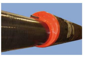
Pull casing end seal over the pipe and fit fastening straps (included).
